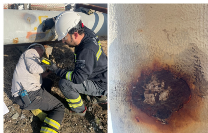
Ultrasonic Thickness Measurement
