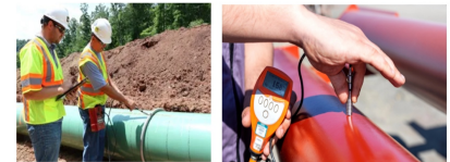
Holiday Test and Paint thickness Measurement
