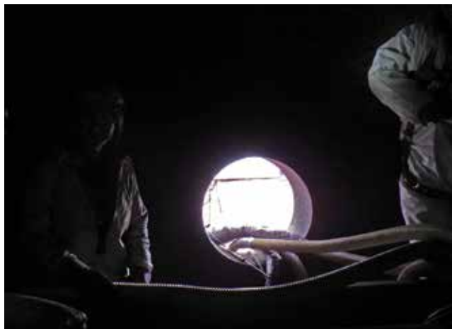
▲ Figure 1. Hazards inside towers include darkness, hoses, and wires. Process inspections often take place during contractor breaks to minimize lost time.
