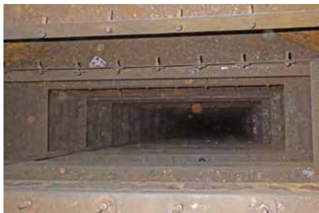
▲ Figure 13. Blind fastening of internal manways is difficult because the clips are not visible to the installer while they are being tightened.
