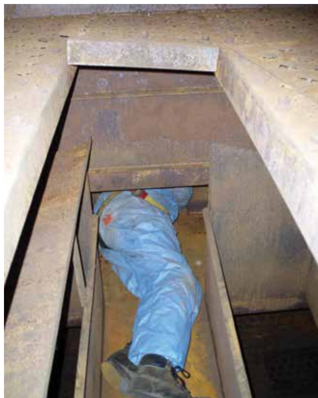
▲ Figure 3. You need a plan for safely entering and exiting a tight space. Body harnesses and other equipment can restrict movement.
