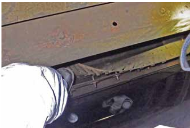
▲ Figure 2. More than one worker or inspector in the same tower section make dropping equipment or dislodging a piece or part even more dangerous.
