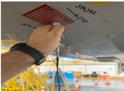
Figure 2 – Corrosion Grid Mapping Data Collection and Analysis
