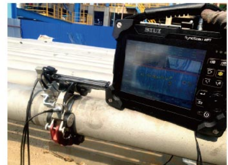
Austenitic weld inspection
