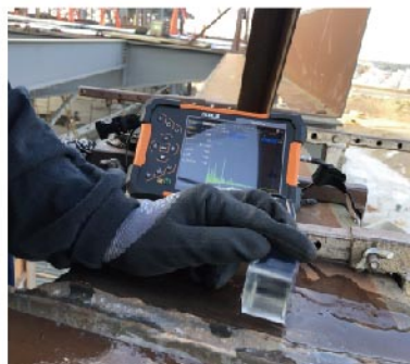
Ultrasonic weld inspection
