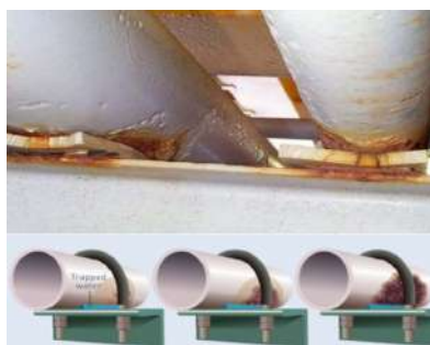
Trapped Water Corrosion
