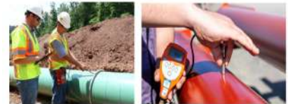
Holiday Test and Paint thickness Measurement
